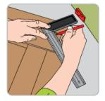
15. Always maintain the expansion gap when the cut is being measured.
